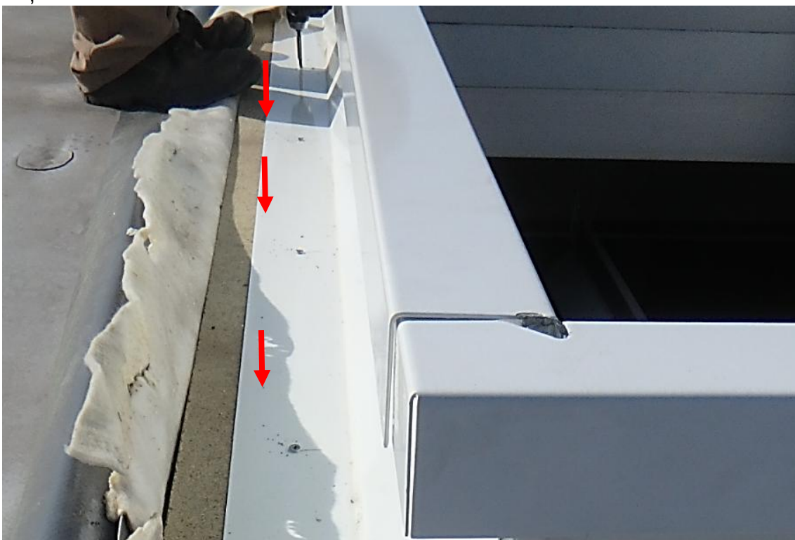
Fig. 30. Connecting the base to the roof with screws.
