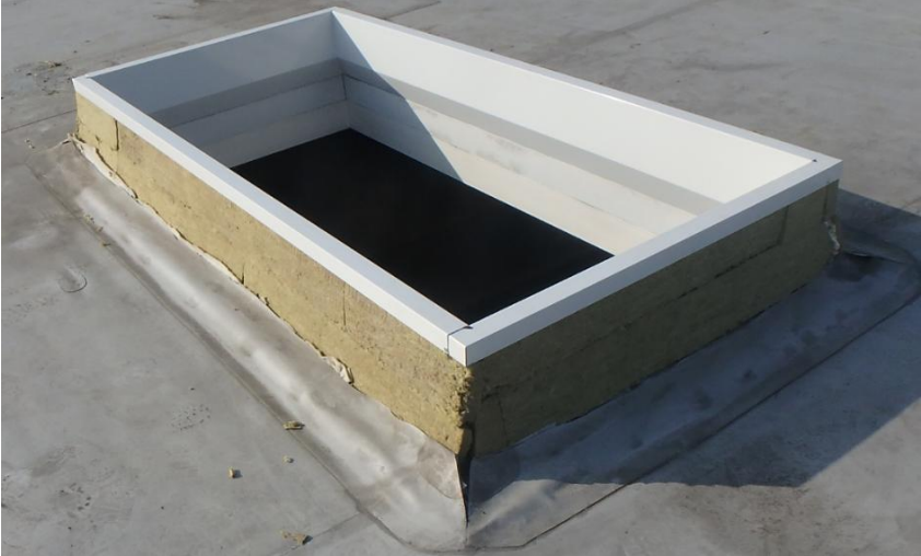
Fig. 31. Insulated base (insulation thickness 50 mm).
